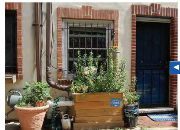
Residential downspout planter installed through the Philadelphia Water Department's Rain Check program. (Photo credit- "Downspout Planter" by Home Science is licensed under CC BY-SA 2.0).
