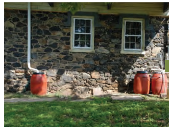
Typical rain barrel downspout connection, private residence.
