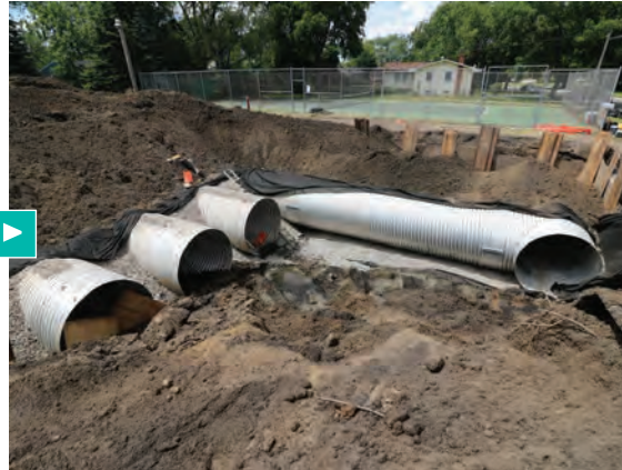
An underground stormwater infiltration system under construction at a park in Minneapolis. (Photo credit-"Infiltration System" by Mississippi WMO is licensed under CC BY-NC 2.0).
