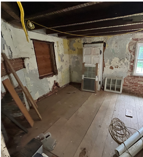
The rear room of the Sexton's House as seen from the doorway between the two rooms. Note the corner fireplace to the left, the boarded window opening, and the missing plaster around the window.
