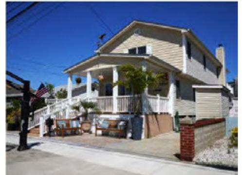
Figure 3-30: Construction of a new building on stilts for the purposes of raising the residence above the flood elevation. The space below the ground floor could be used for parking.
